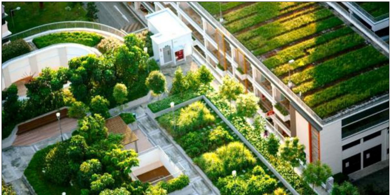
Figure 5 Green Roofs to Enhance Thermal Performance and Their Adaptability in Texas (Bing (n.d.), 2024)
