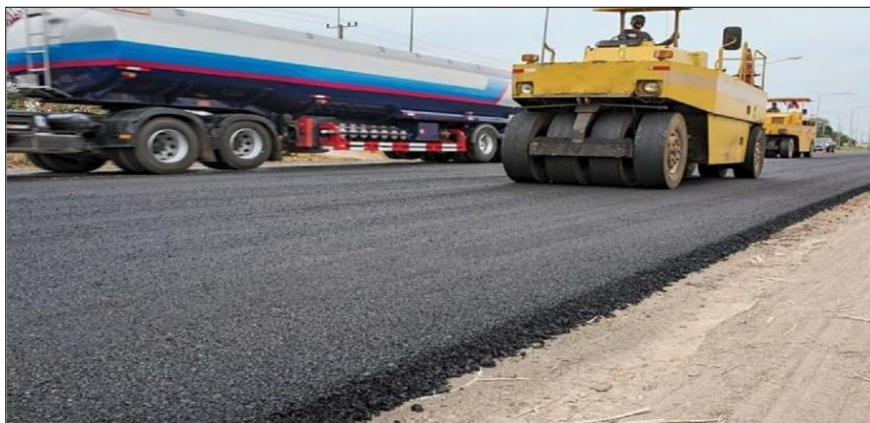
Figure 3 Paving Road using Waste tyres
